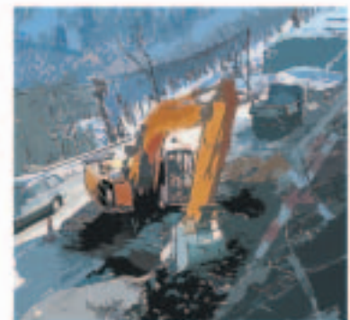
Road widening construction
